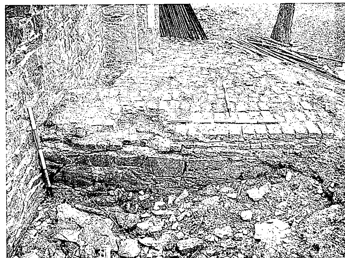
Figure 9. The north door double staircase base. It reflects the façade of the house in its stone base and brick paved surface. It is not bonded to the house.
