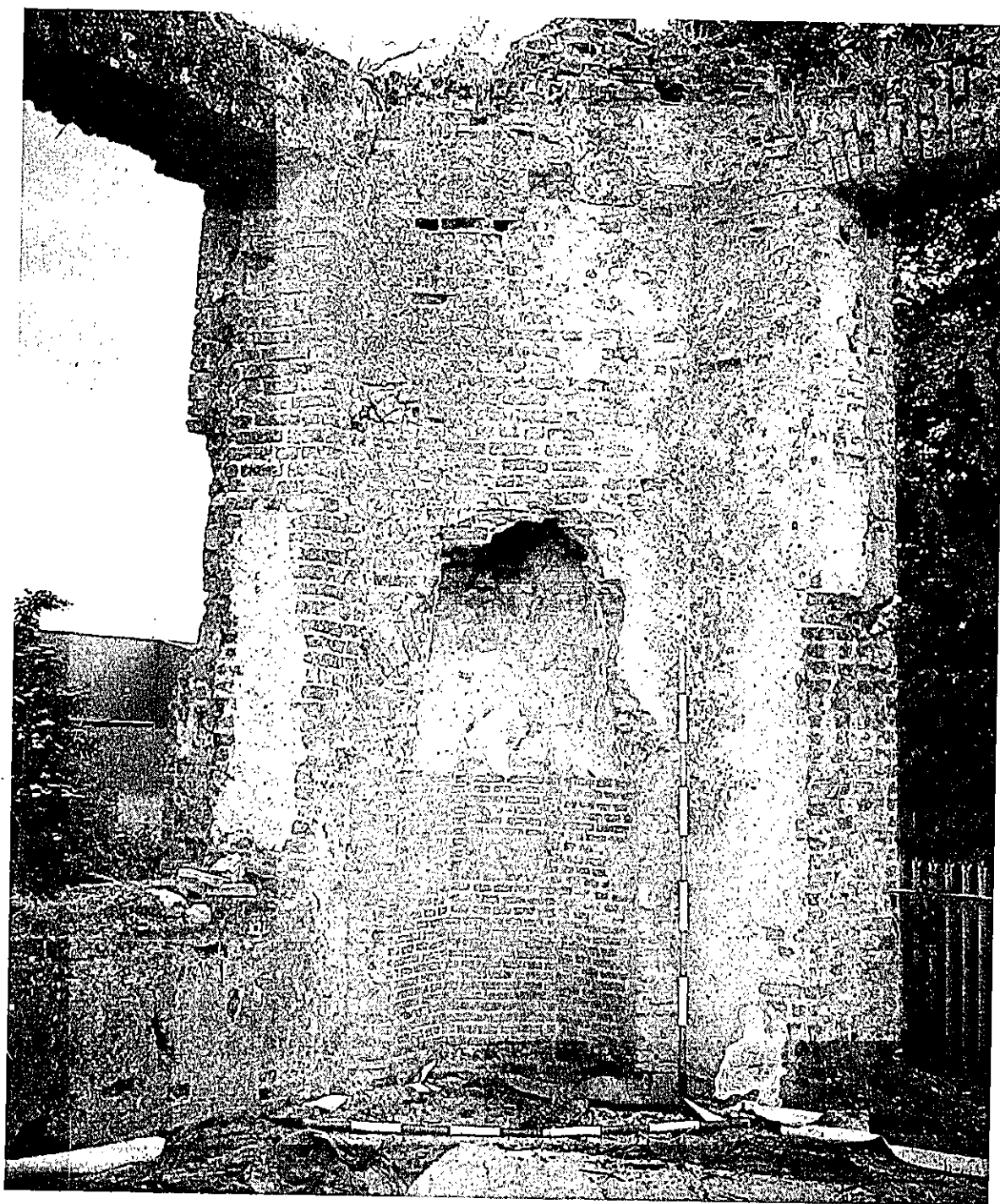
Figure 20. Southeast corner fireplace. Note the remains of an arch to the top left of the fire opening and the large narrow Dutch-style window to the right with flat arch and transome notch about 2m up.
