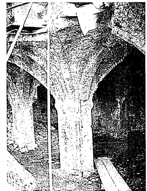
Figure 24. East wing basement with two central supporting columns. Note the moulded brick and rib vaults.
