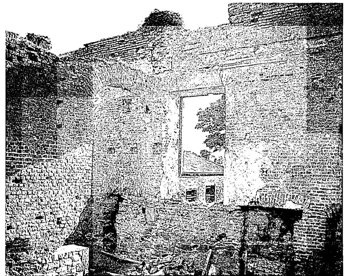
Figure 16. West end interior of house. Note the arch, floor joist notches and the peculiar window heights that are indicative of a staircase.
