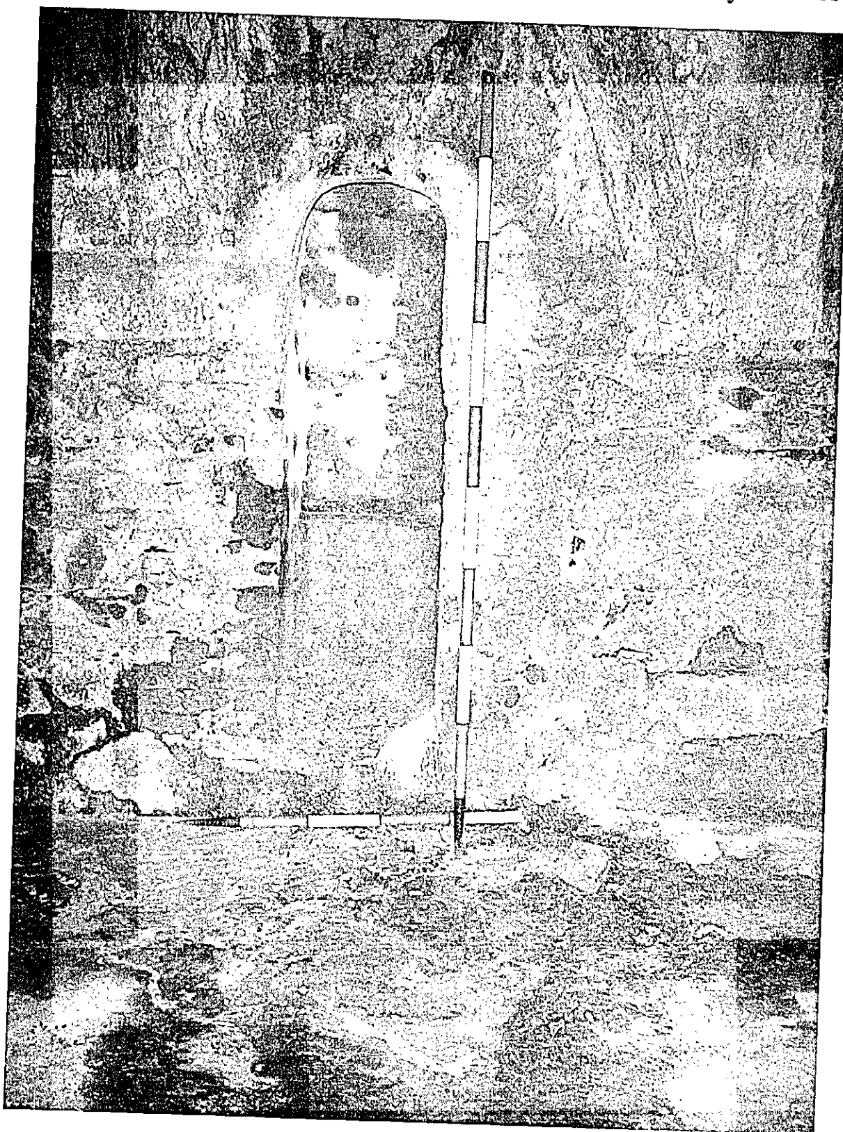
Figure 25. Basement vent shaft. Note the shelf cut into the vent about 70cm up, the brick surround and the shallow trenches leading out straight from the shaft and to the right.
