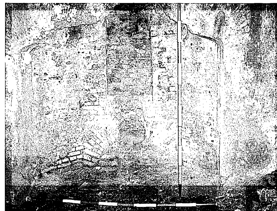
Figure 21. East wing west basement fireplace. Note the stone surround, the arch cut into the surround and the small red back panelling bricks.
