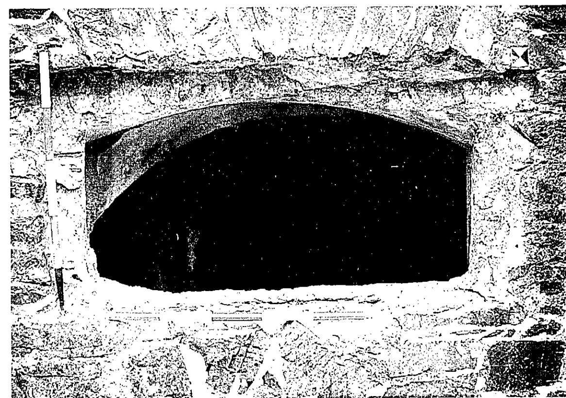
Figure 11. North wall splayed basement window. Note the flat arch of vertical bricks.
