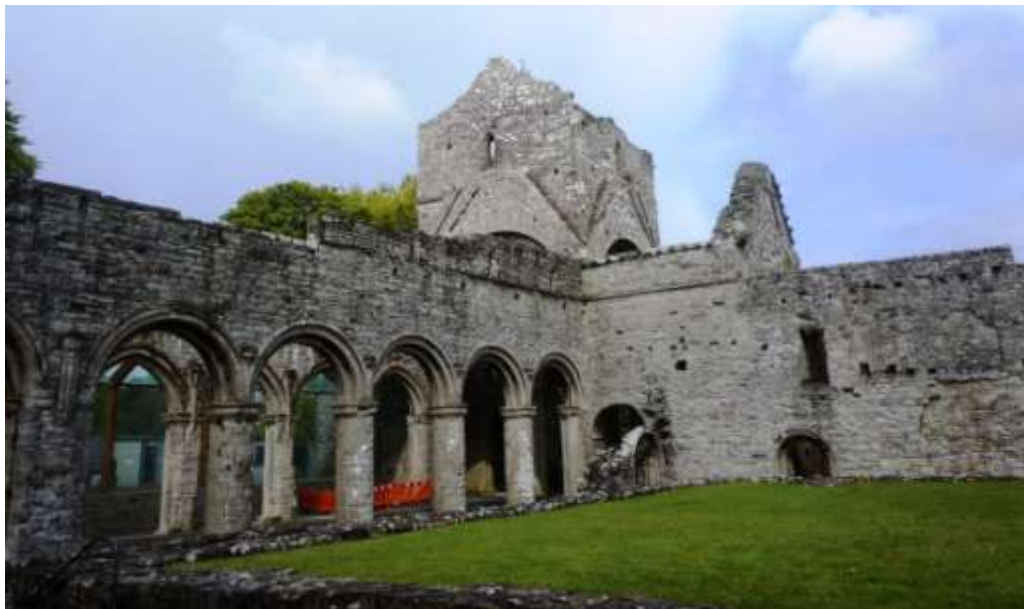
Boyle Abbey showing the extent of the structure and part of the new wood and glass structure on its north aisle.
